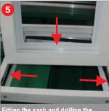
Fitting the sash and drilling the mounting holes in the frame
